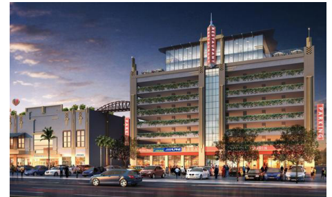
(Osman Baig) Mango's parking garage . Developer Wallack Holdings LLC has added a new feature atop its $20 million, seven-story public parking garage on International Drive — a glass-enclosed eatery space.
